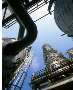
Methanol Plant 1MMT/year
